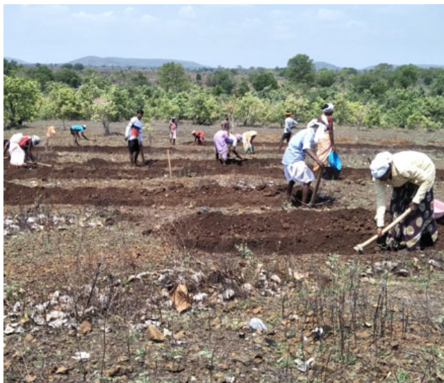
Restoration work at the Commons
