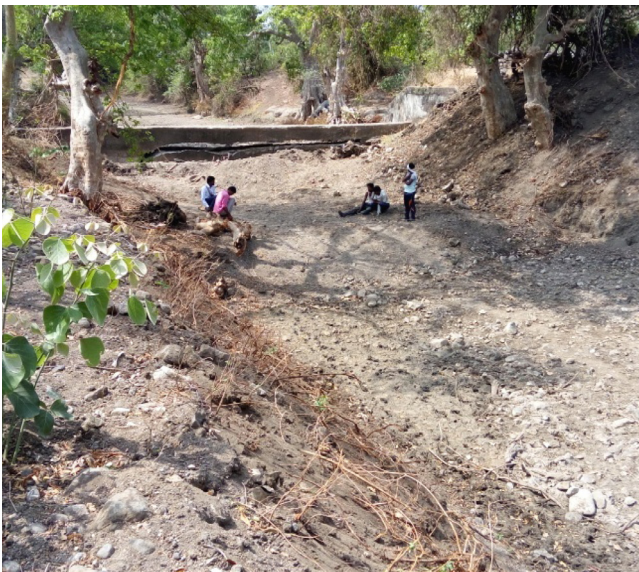
Jarur Hiwardhara Nala before the restoration work began.
