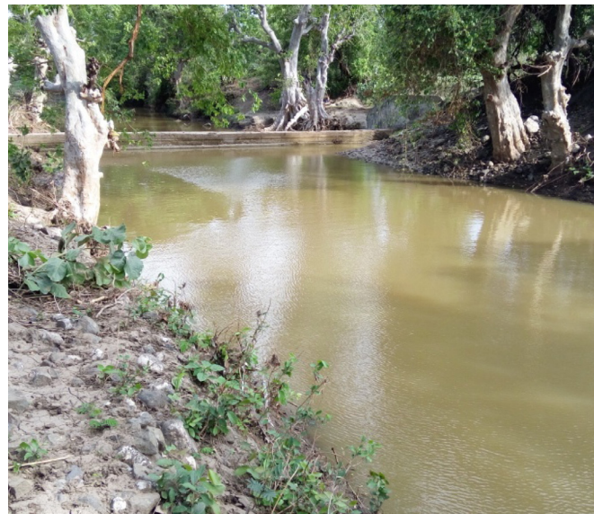
Jarur Hiwardhara Nala after the restoration work was completed.
